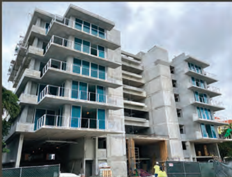
Construction status, January 2018
