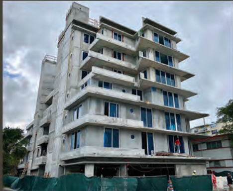
Construction status, January 2018
